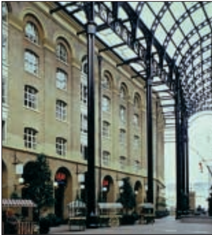
Hay's Galleria, offices with a public link through the galleria and active uses on ground floor
