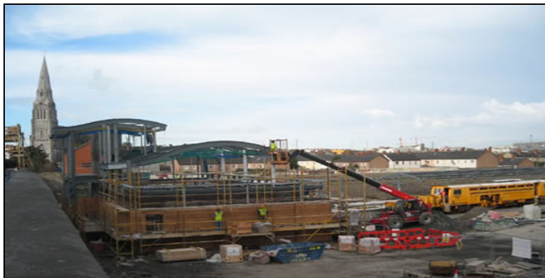
Figure 5.4: Docklands Rail Station Construction
