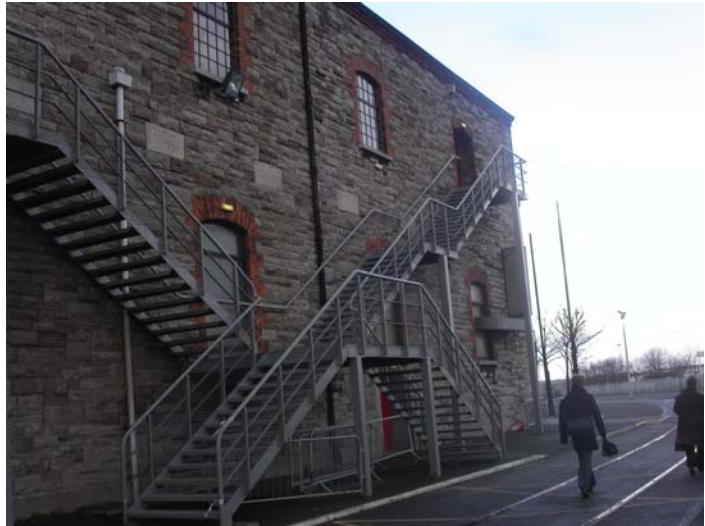
Typical fire escape staircase arrangement on east elevation
