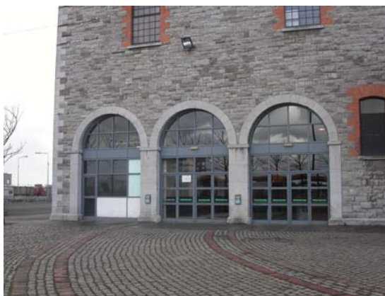
Group of three arched openings on the north elevation with new cobbled apron in the foreground
