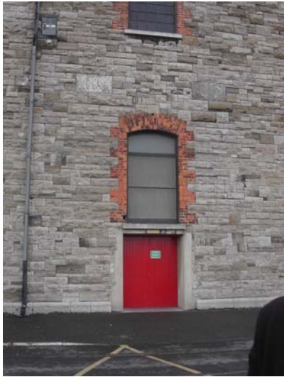
Altered opening and ground floor fire exit on east elevation
