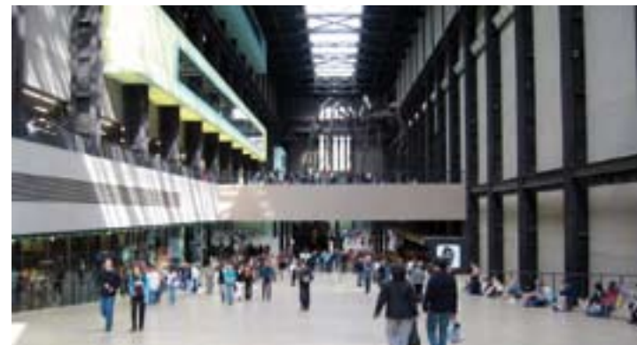
Example of a conversion of a former Power Station: Tate Modern, London
