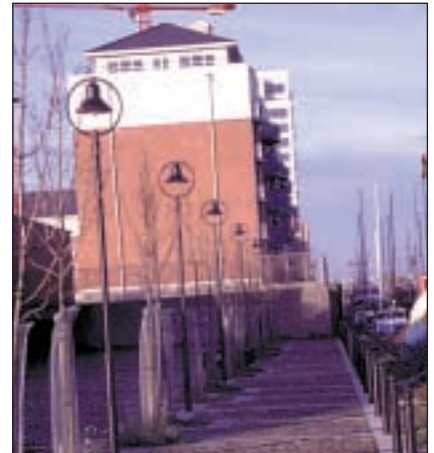
Existing quayside link to be extended
