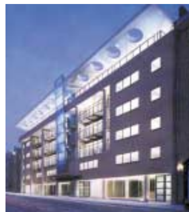
Quality office development
