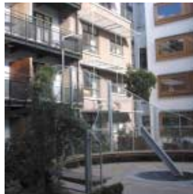
Recent high quality residential development
